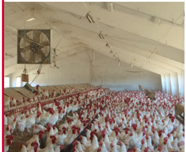
Figure 96 Circulation fans in an open-sided/naturally ventilated house.
