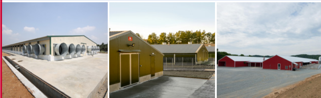
Figure 9 Houses with a low biosecurity risk showing concrete areas and no vegetation around the immediate perimeter of the house.
