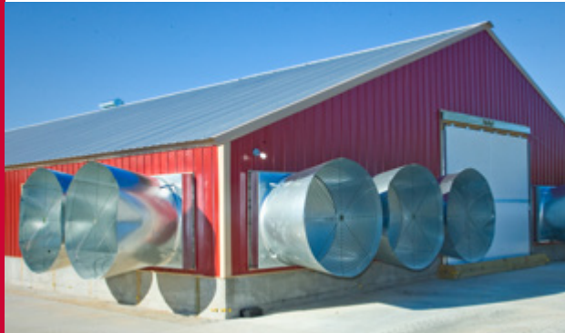
Figure 107 Example of a typical tunnel-ventilated house.
