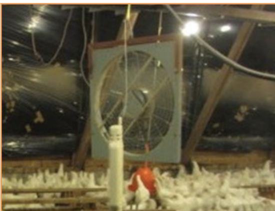
Figure 6: Example of a circulation fan.
